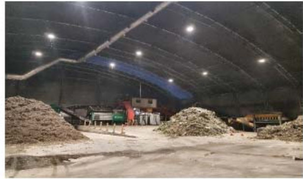
Figure 3-9 Example of central ductwork for extraction of process air from the building
