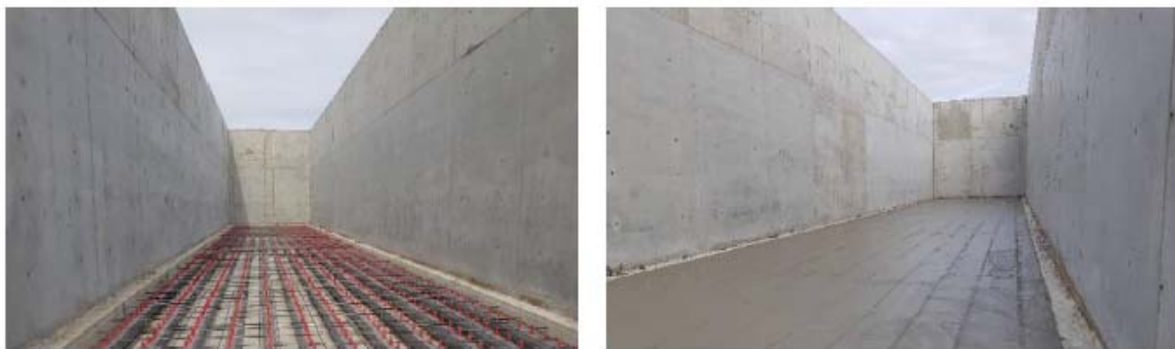
Figure 3-6 Construction of the spigot floor utilised for the composting tunnels
