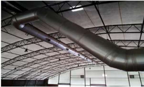
Figure 3-9 Example of central ductwork for extraction of process air from the building
