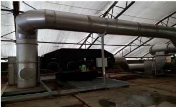
Figure 3-10: Example of humidifier and ductwork
